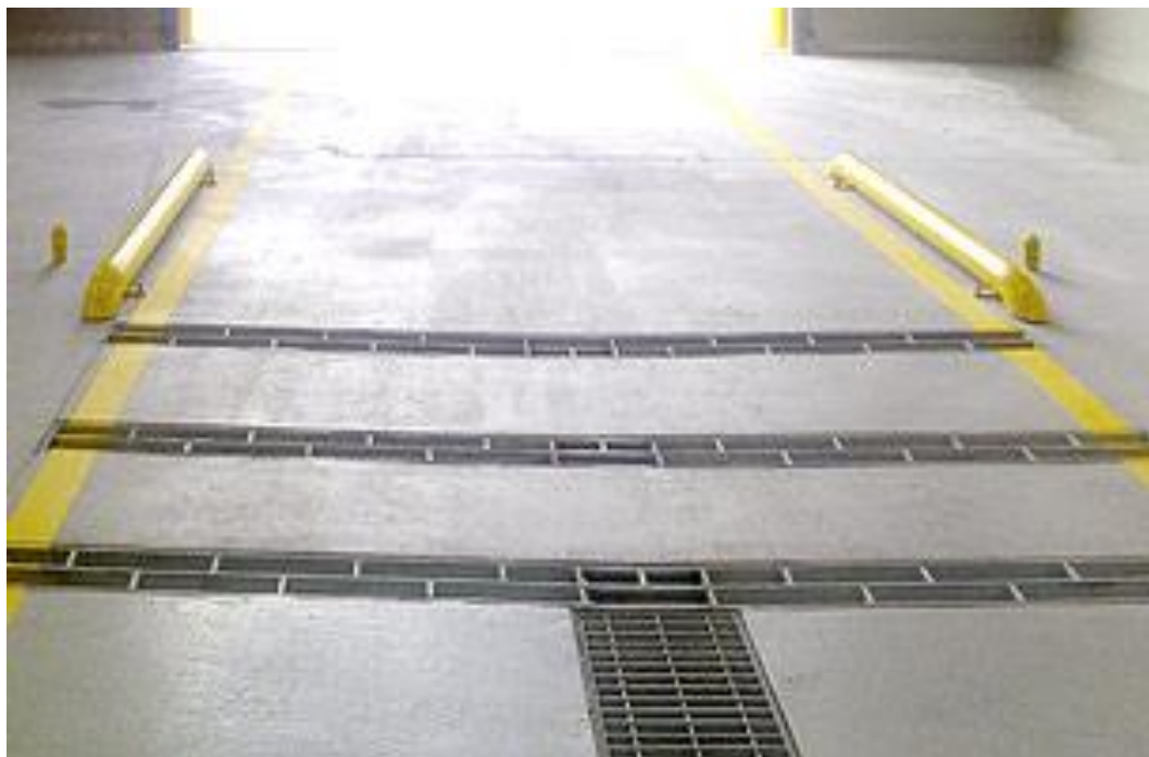
Figure 7 Indicative Wheelwash (Source: HARTEX)
